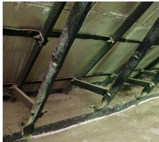
Figure 10: Base detail showing wall plate (Heres 2012)
