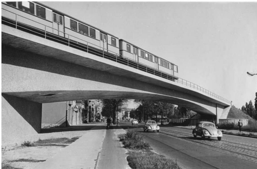
Figure 1: The Seidelstraße Bridge, just after completion in October 1959.
